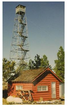
LS-40 Metal Aermotor: Criss-Cross Stairs, 7'x7' Cab
